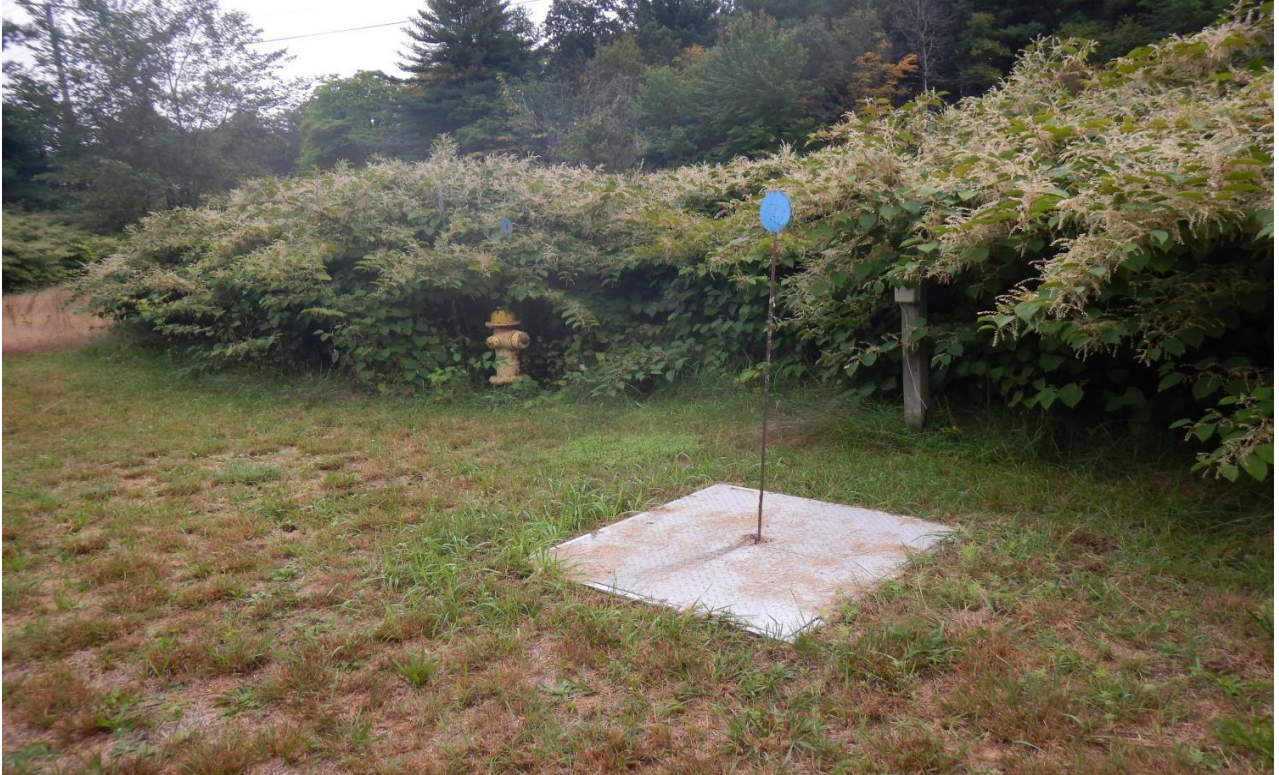
Photo 7: Maintenance access hatch with electrical box and fire hydrant within parcel limits.
