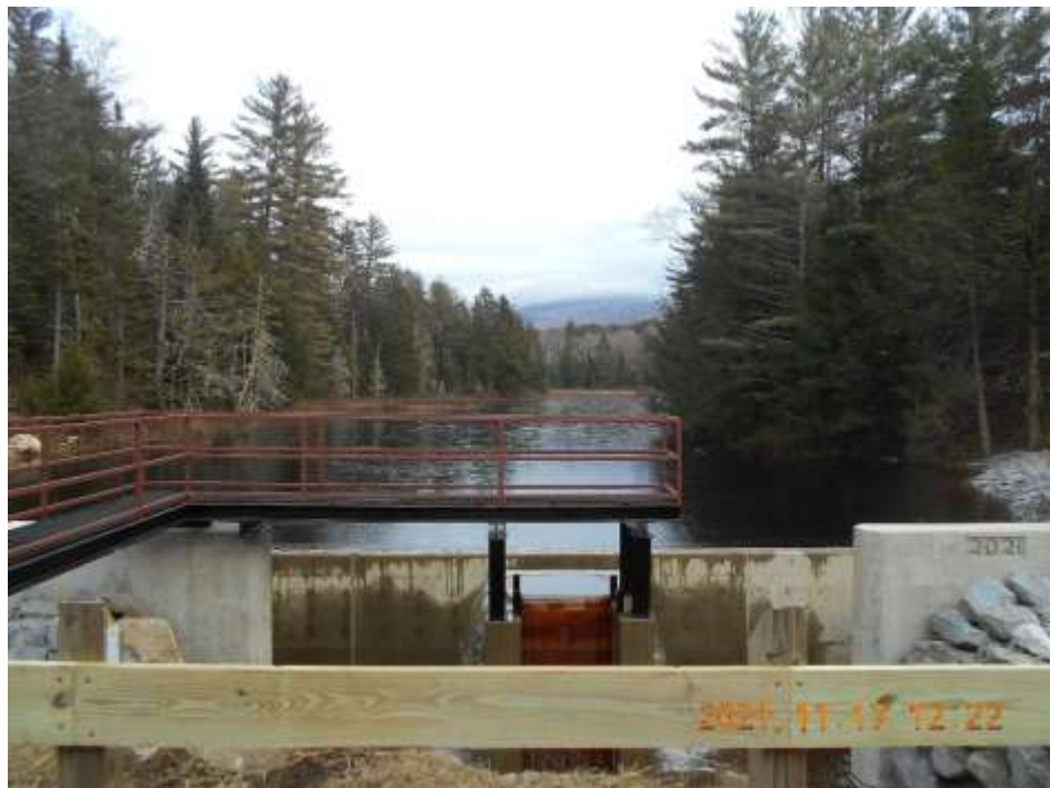
Photo 6: New Weeks Crossing dam looking northeast at Pond 11/2021.
