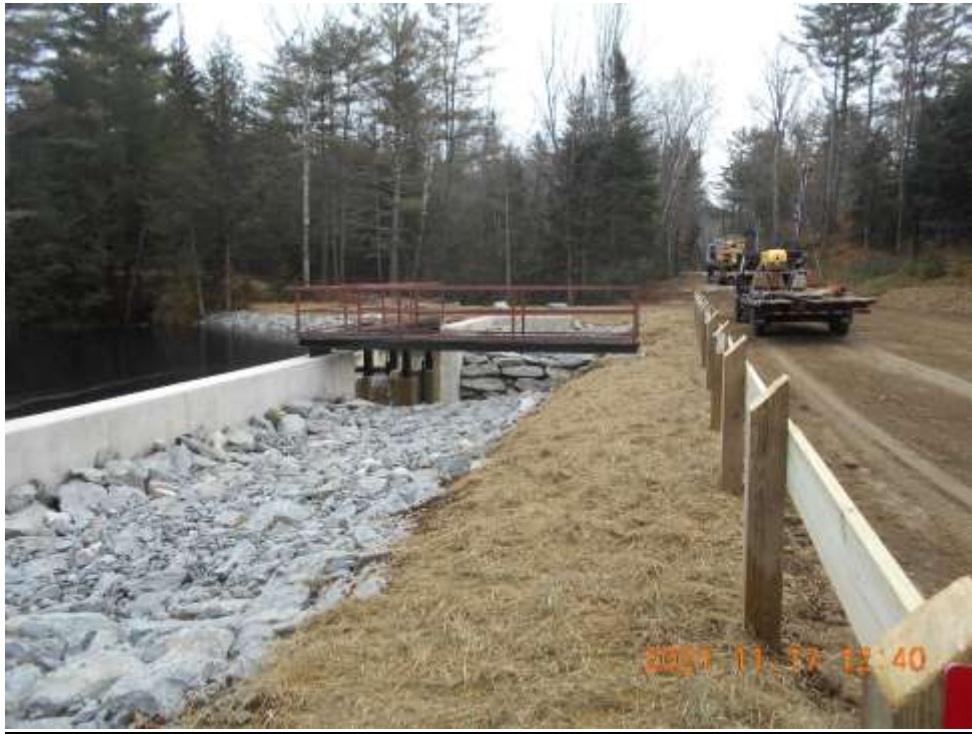
Photo 5: New Weeks Crossing dam looking southeast 11/2021.
