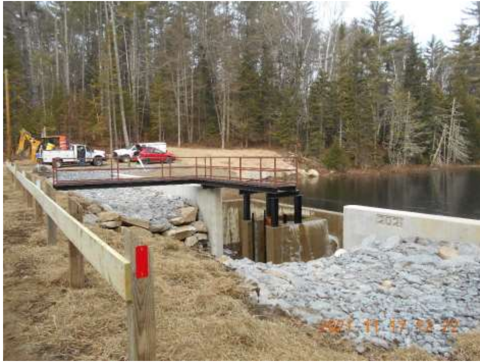
Photo 7: New Weeks Crossing dam looking northwest at pond 11/2021.
