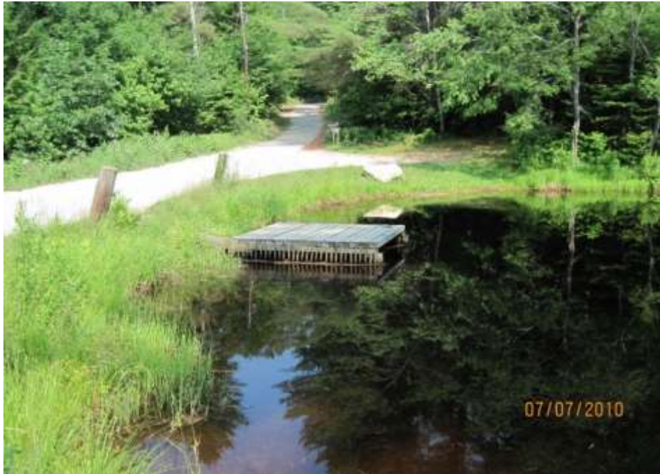
Photo 1: Weeks Crossing Dam looking northwest before failure. 7/2010
