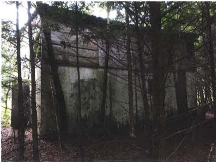
Looking south at the back of ancillary building.
