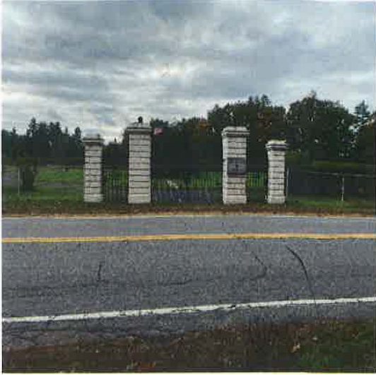
Parcel #: 21 columns Station: 527+50 Rt
