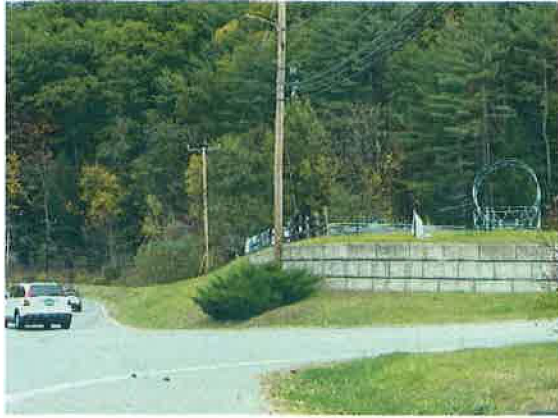
Parcel #: 5C retaining wall Station: 515+50 Lt.
